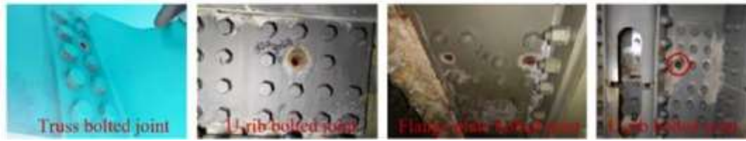
Fig 2.3 Typical Bolt dropping (source: Chuang Cui 2024)
