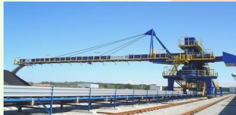
Figure 1. Limestone Luffing Stacker Machine at Cement Plant Site
