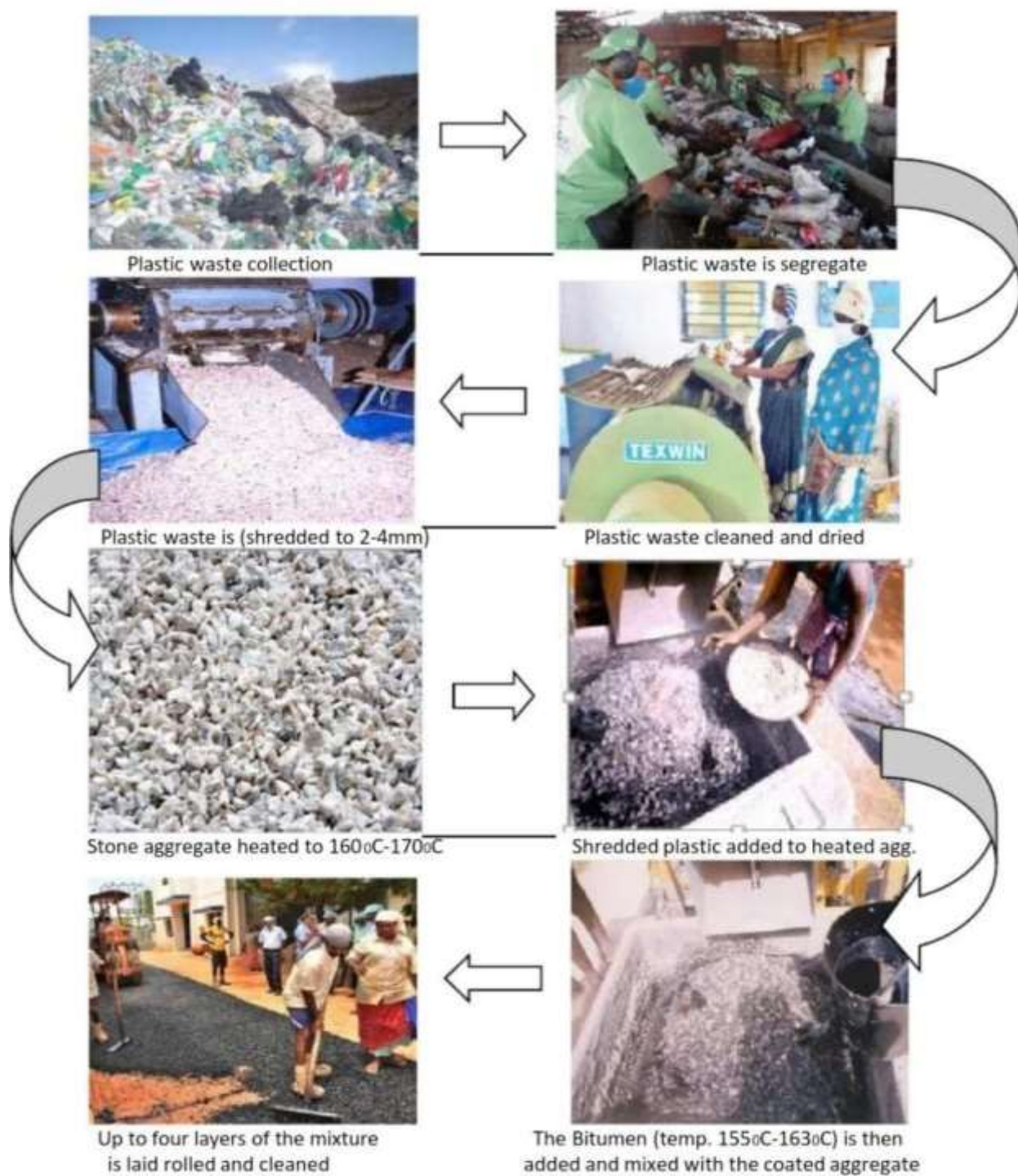
Fig. Construction Process of Plastic-Coated Bituminous Road
